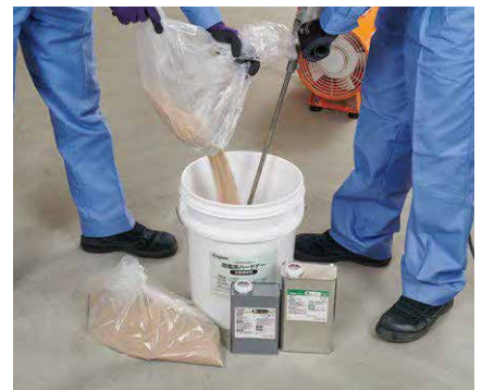
Mix in aggregate (always use a mixer)
