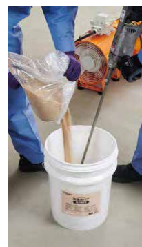
(3) Mix in aggregate (always use a mixture)
