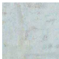
MBE-511 LN 38 Wall Concrete (S) ★ REAL
