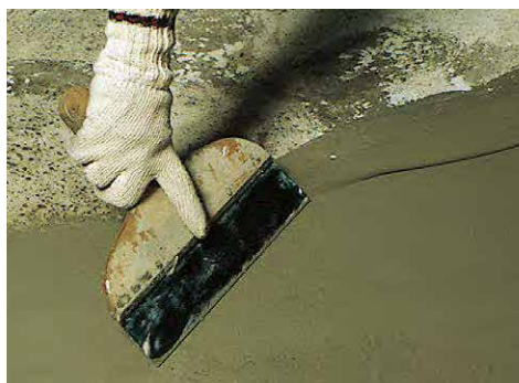
Apply to entire surface using a flooring spatula.
