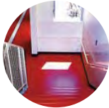
U-MANITY Installation site No. 1
