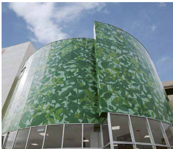
Subfloor: Extruded cement panel Vinyl chloride film for external use Full-color printing
