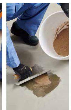
(4) Apply using plastering brush, pushing in (lower than level of subfloor)
