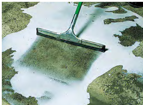
Apply to entire subfloor surface using a squeegee, roller brush, etc.
