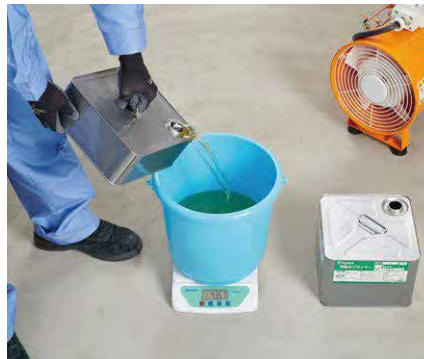
Measure solutions A and B using a scale and combine (by weight)
