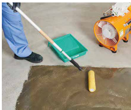
Apply using a roller brush. Always use ventilation fans (explosion-proof type) while applying.
